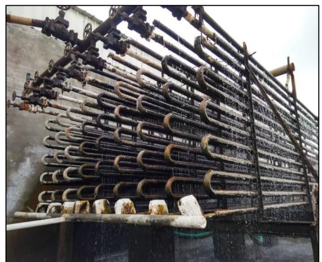
Fig. 3 Construction of Atmospheric Condenser
